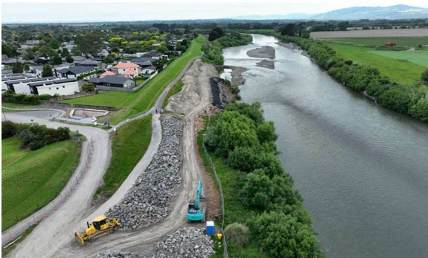
Figure 12: Photos in two flood protection upgrades completed as part of the Climate Resilience work programme. Above: rock armouring at Te Matai Road, Manawātū River. Below: Albert Street Palmerston North.
