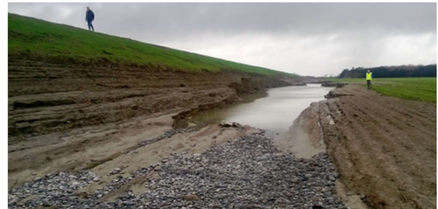
Figure 8: Inspection of a stopbank damaged during a storm event. Climate change is likely to increase the amount of asset inspection and repair work required.
