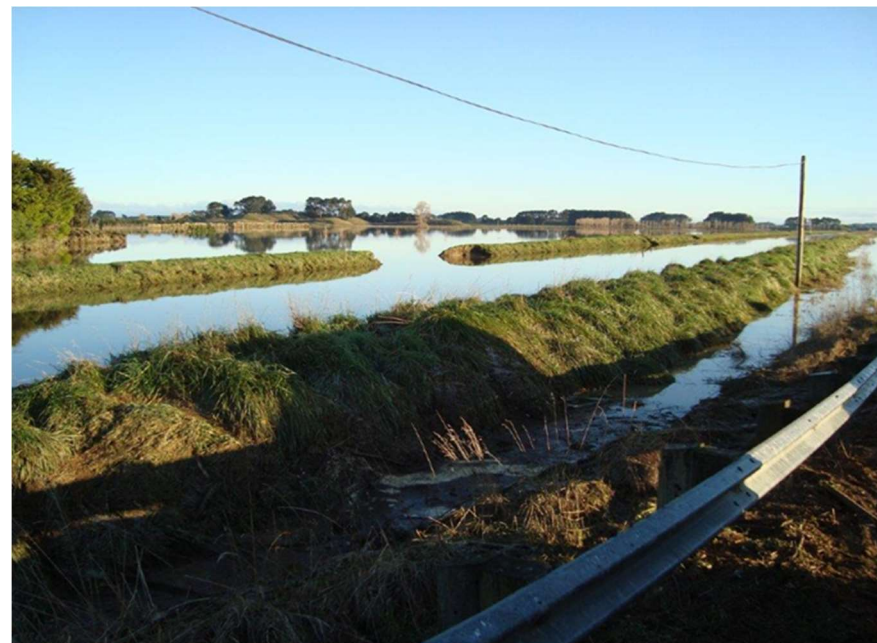
Figure 19: Example of asset failure. Stopbank breach in Sluggish Main Drain in the Te Kawau Drainage Scheme during the 2015 flood event.
